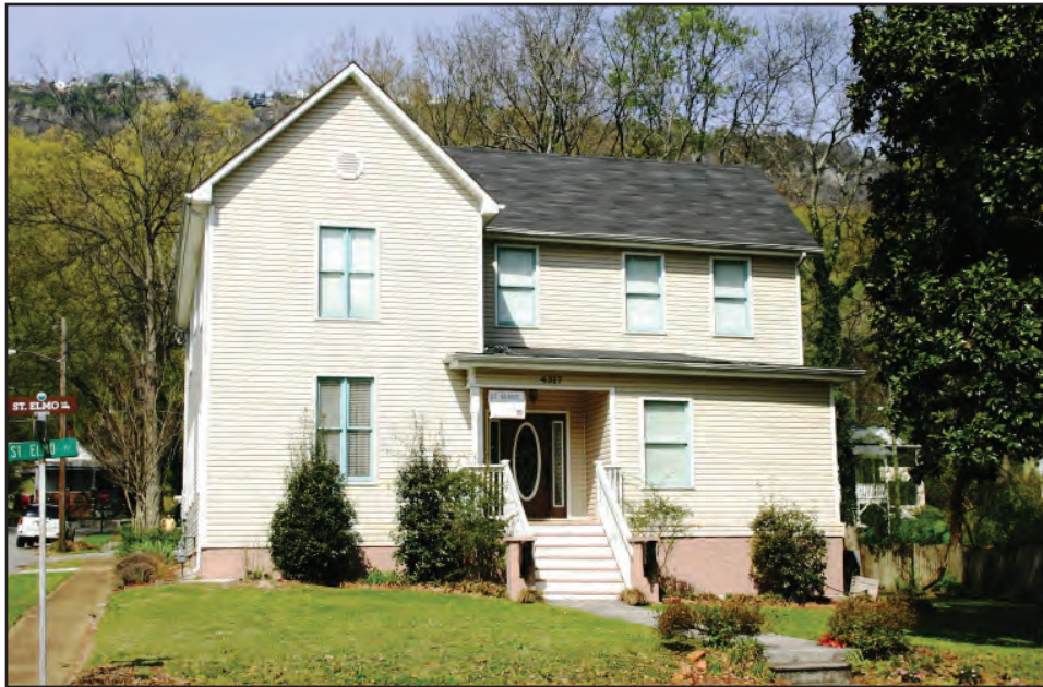
The gable roof of this vernacular farmhouse has a timeless appearance with its attractive, symmetrical shape.
