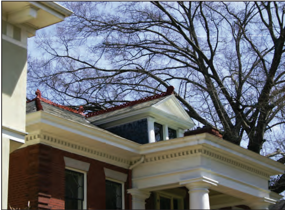
The metal coping on this house is consistent with the visual character of the neighborhood.
