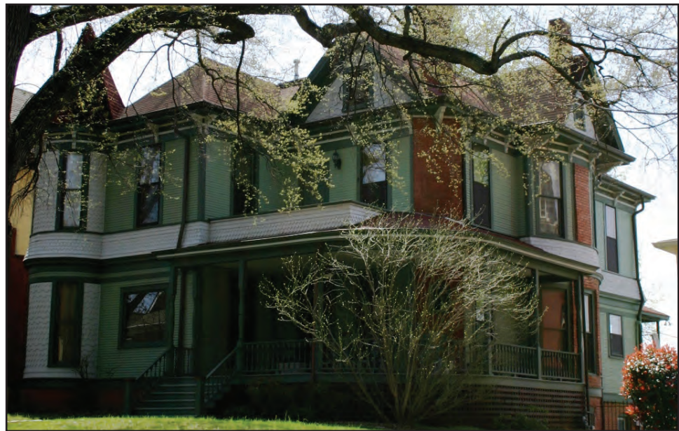
Historic wood siding should be maintained and preserved.
