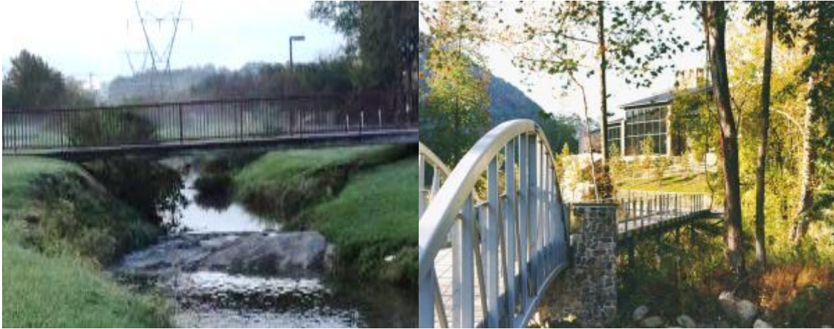
Figure 5.2.1.1-4. Bridges over valleys to facilitate access.
