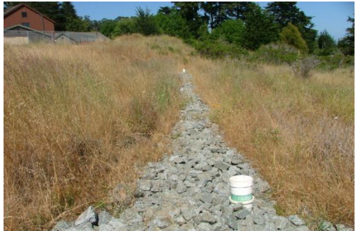
5.2.1.2-3. Level spreader along contour of slope.
