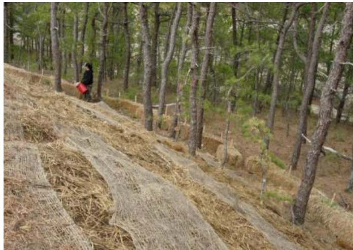
5.2.1.2-7. Steep slope erosion management installation.
