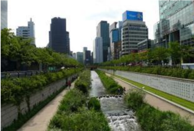
Figure 5.2.3-5. Urban Example – Cheonggyecheon River Restoration Project.
