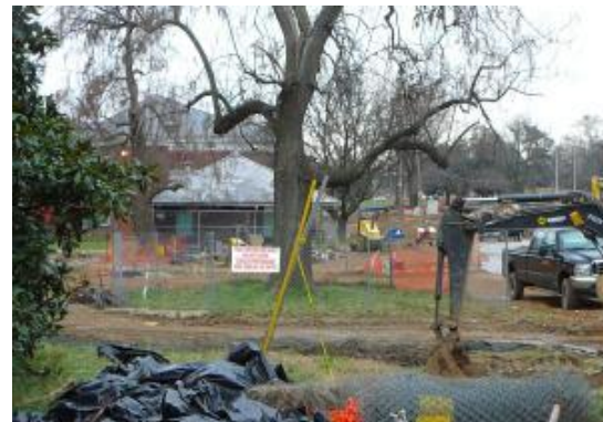
Figure 5.2.4.1-2. Tree protection fence with sign.
