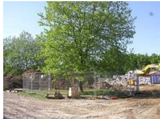
Figure 5.2.4.1-1. Tree protection fence.
