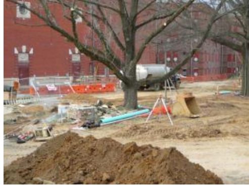
Figure 5.2.4.1-9. Do not stockpile in root zone.
