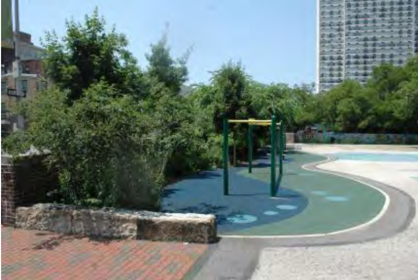
Figure 5.3.4-5. Institutional bioretention area at an urban schoolyard (adjacent to porous rubber play surface).
