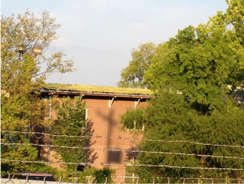
Figure 5.3.8-5. Chattanooga green roof at the Crash Pad.
