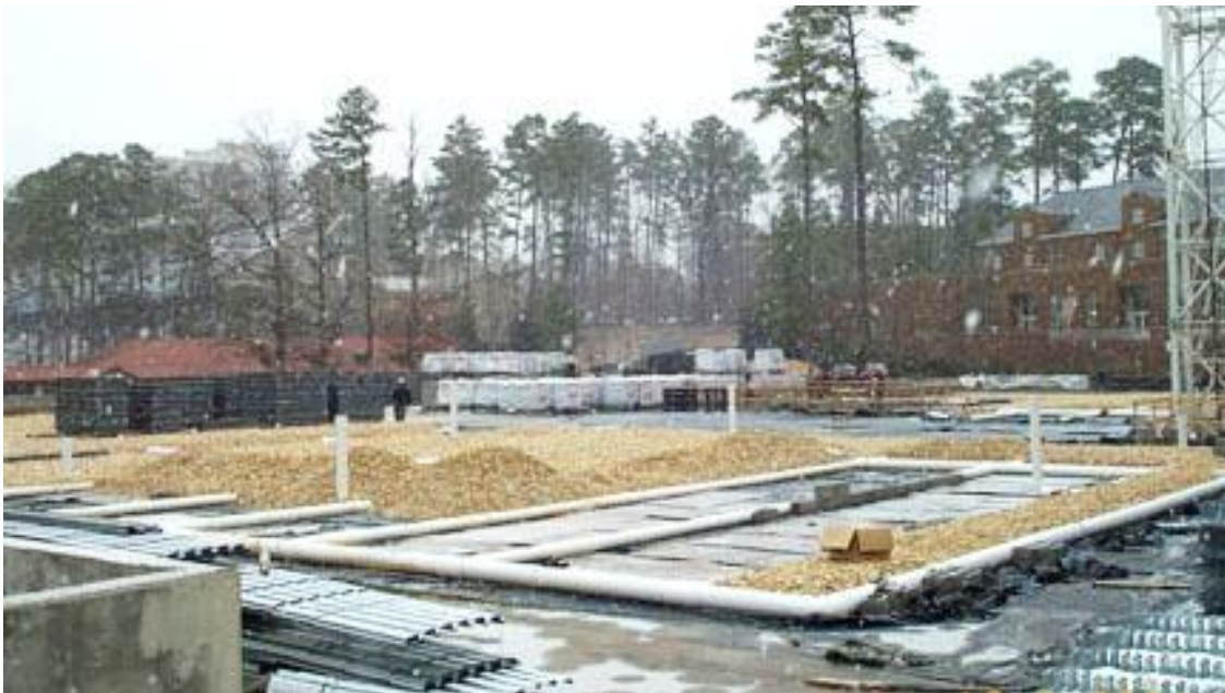
Figure 5.3.8-9. Installation of drainage layer beneath intensive green roof.
