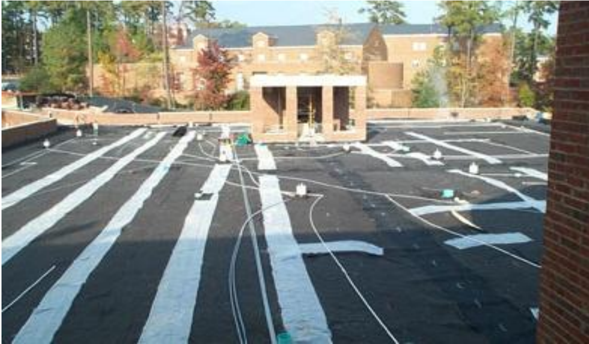
Figure 5.3.8-10. Geotextile and root protection.
