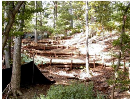
Figure 5.4.1-7. Log check dam installed.
