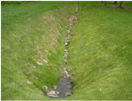
Figure 5.4.1-9. Avoid straight, uniform cross-section grass swales where possible.
