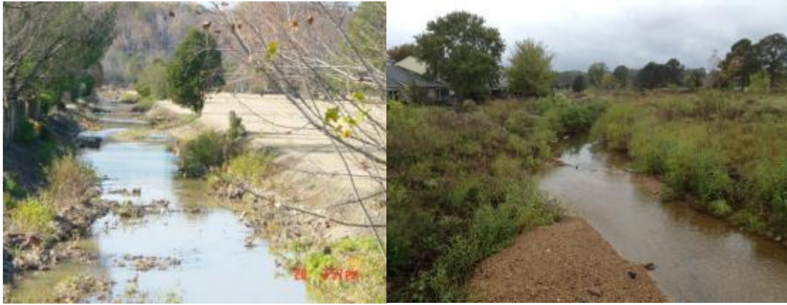
Figure 5.4.1-4. Hickory Valley CC (now “First Tee”) restored stream channel (before and after).
