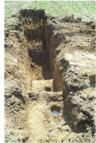
Figure C-1. Soil test pit.
