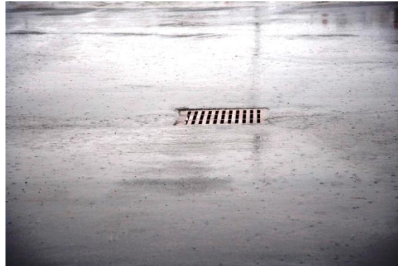
Figure 1-3. Typical impervious surfaces in Chattanooga generate runoff nearly every time it rains, conveying pollutants to streams.
