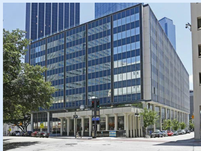
The Mayflower in Dallas, utilizing TIF financing, contains 215 units of housing, 43 of which are affordable.
