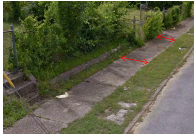
Sidewalk Cross Slope, as depicted by arrows
