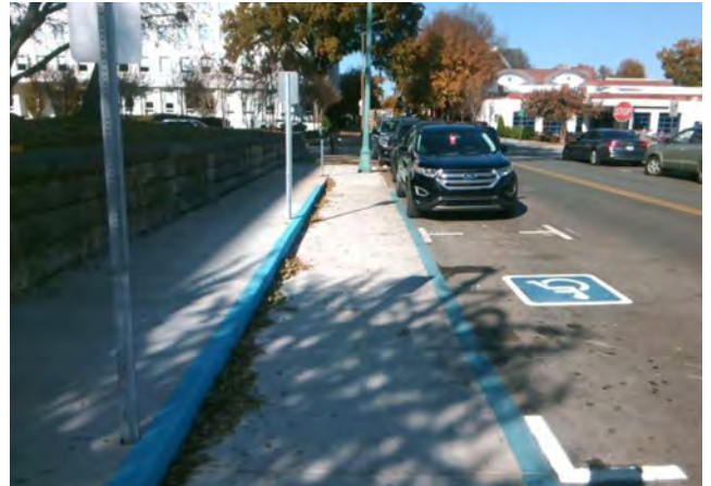
Accessible Parking Spaces
