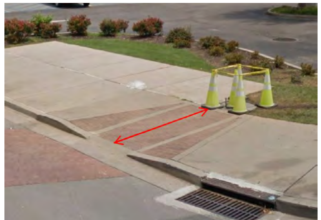
Curb Ramp Run Slope
