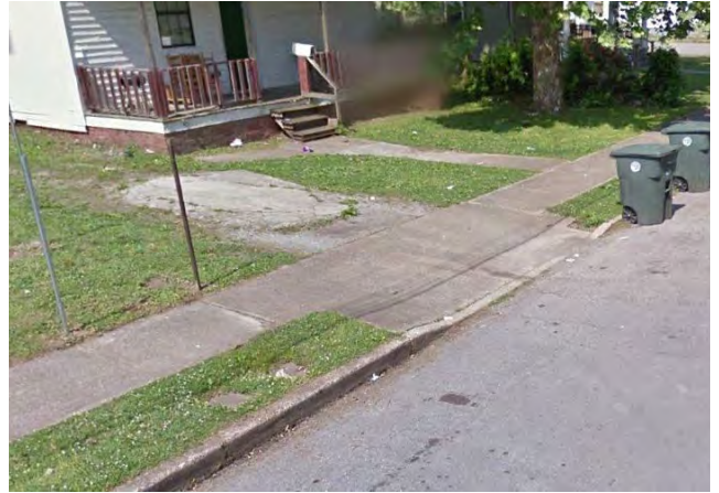
Sidewalk built through a driveway
