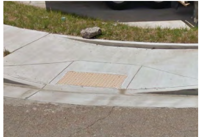
Curb Ramp Detectable Warning Surface
