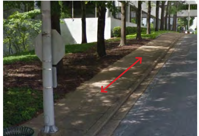
Sidewalk Run Slope, as depicted by the arrow
