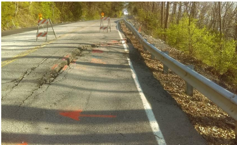
Slope failure
