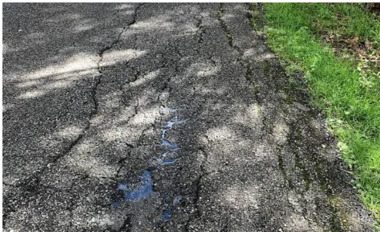
Base failure
