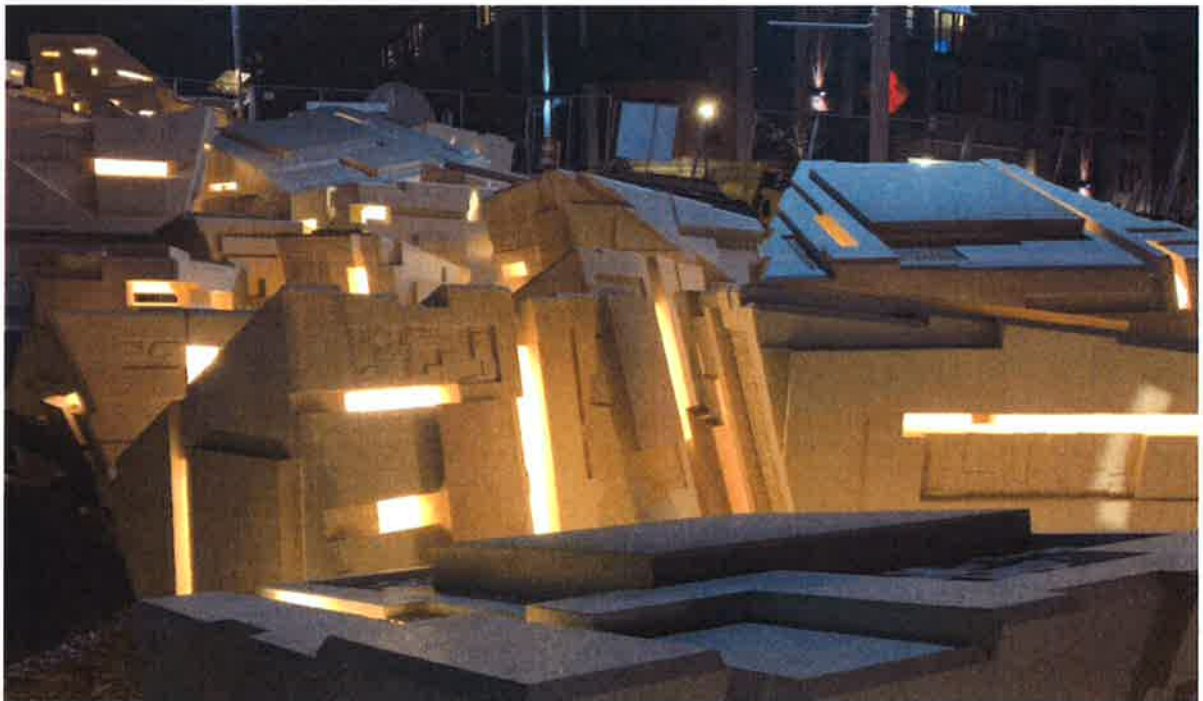
Evening photo during construction in late December 2020
