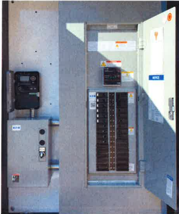
Left: contents of the new electric enclosure. (a) Electric panel and circuits at right, with (b) surge protector above (black square). (c) Accent lights power supply at the bottom left, with (d) controlling timer above.
