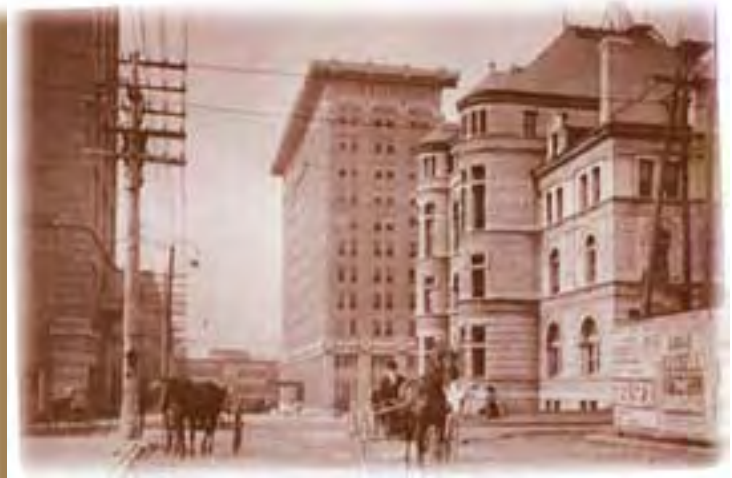
In the right foreground you can see the construction site for City Hall, with the Custom House and the Hotel Patten in the background.
