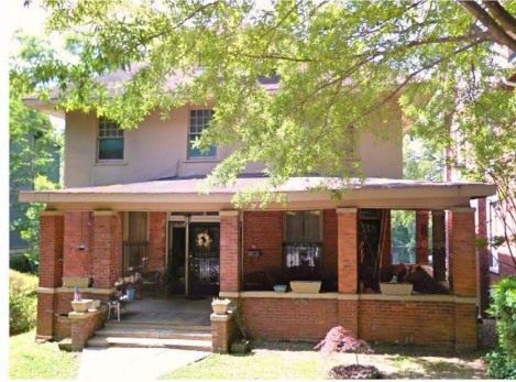
Porch prior to demo, shows brick knee wall
