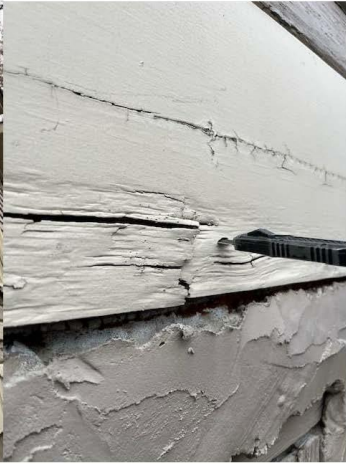
4507 Tennessee Avenue – ROTTED WOOD AT EXISTING HISTORIC SIDING ** SOUTHERN FAÇADE **
