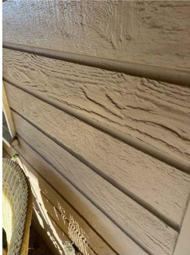
4507 Tennessee Avenue – DETAIL VIEW OF NON-HISTORIC SIDING (AT BACK PORCH AND REMOVED, AT FRONT PORCH REQUESTING
