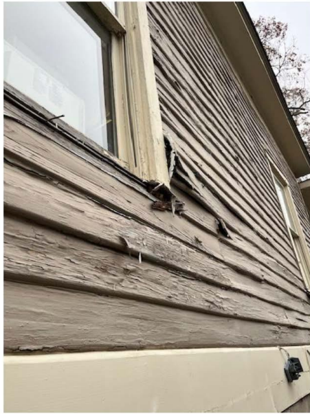
4507 Tennessee Avenue – ROTTED WOOD AT EXISTING HISTORIC SIDING ** SOUTHERN FAÇADE **
