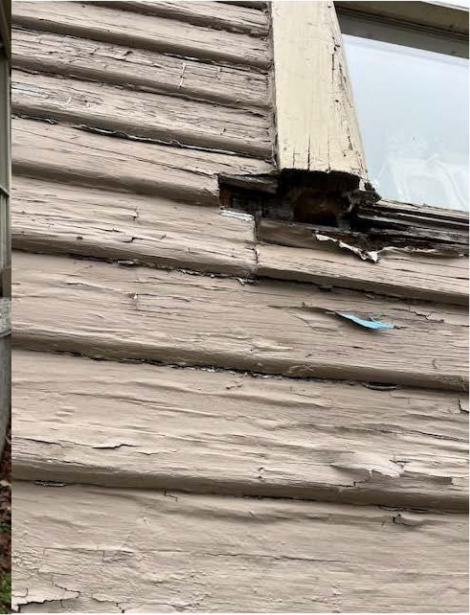
4507 Tennessee Avenue – ROTTED WOOD AT EXISTING HISTORIC SIDING ** SOUTHERN FAÇADE **
