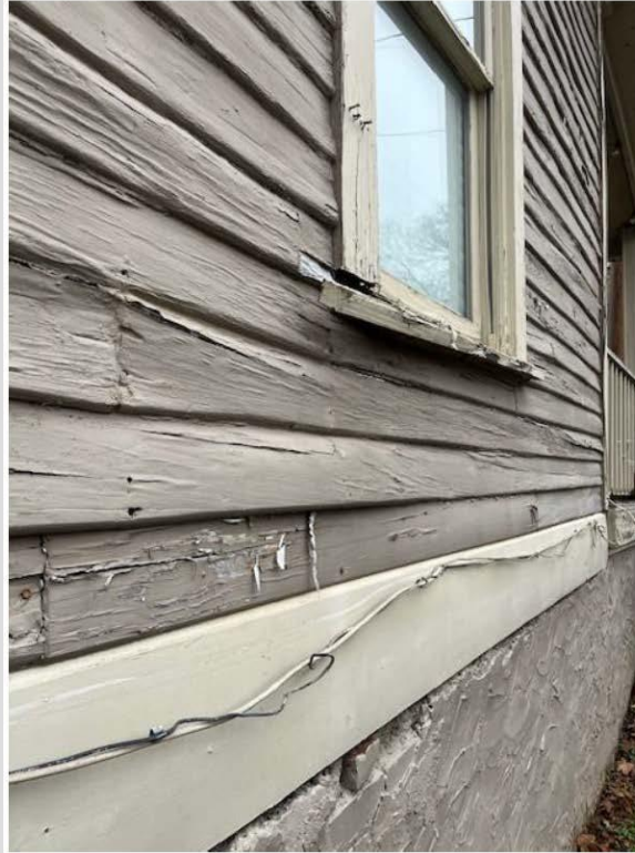
4507 Tennessee Avenue – ROTTED WOOD AT EXISTING HISTORIC SIDING ** SOUTHERN FAÇADE **
