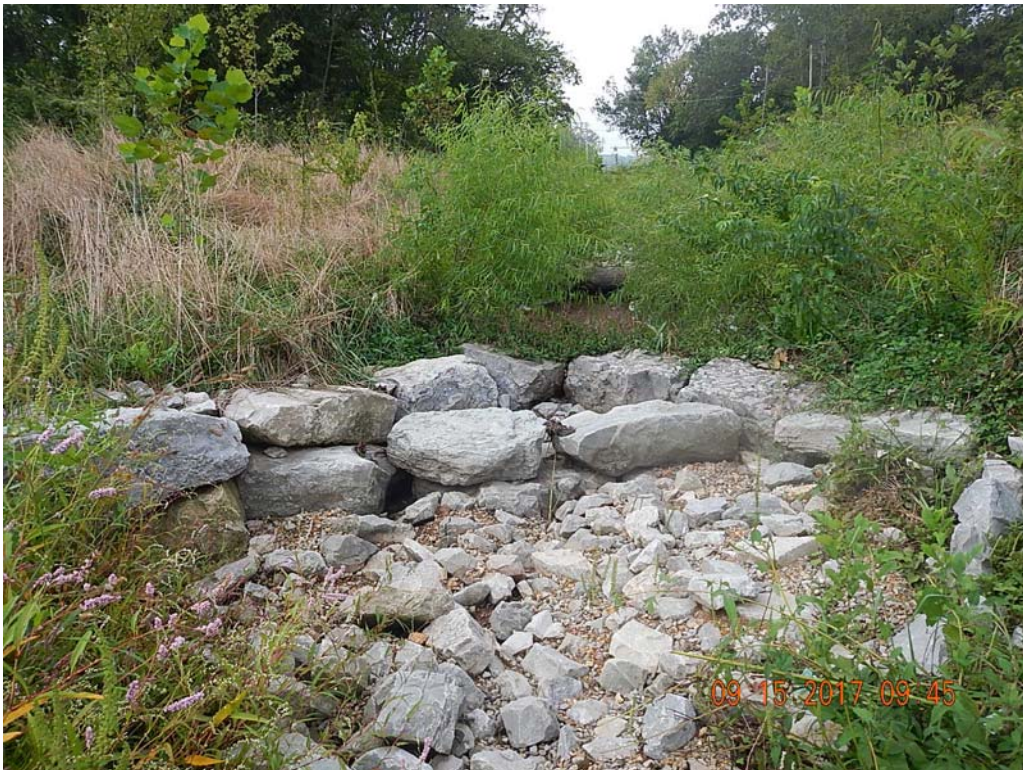
Figure 12 Upstream view of unnamed tributary showing stable structures
